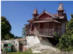
Outbuilding, damaged by the 2010 earthquake, and barbershop kiosk; Léogâne, Haiti
