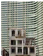
Partially demolished building with Edificio FOCSA in the background, Vedado neighborhood; Havana, Cuba
