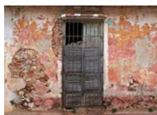
Facade; Trinidad, Cuba
